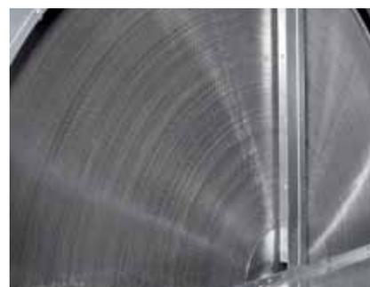
High-efficiency exhaust air plug fans. The fan speed is independently controlled by frequency inverters directly connected to the Pro-Dialog+ control inside the rooftop unit.
